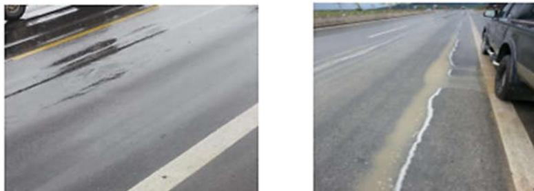
**Fig. 1.** The ruts of wheel tracks on National Highway 1, section Vinh - Ha Tinh [1].
