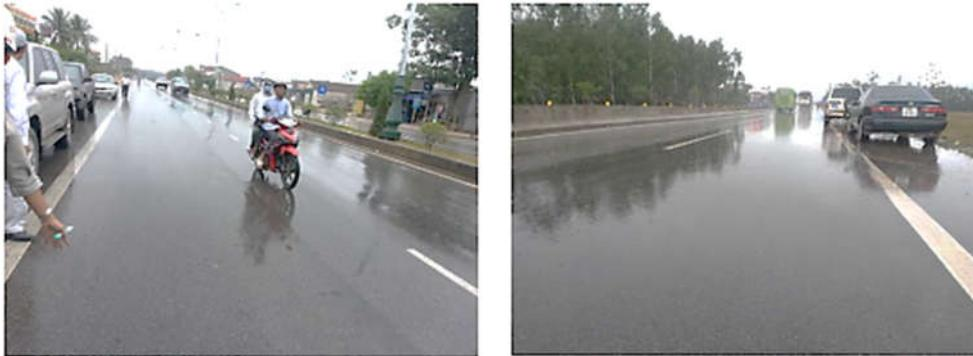
**Fig. 3.** In the same section of the route, there are still parts of the road that do not have rutted wheel tracks (National Highway 1 section of Vinh - Ha Tinh).
