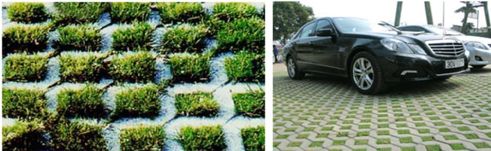
**Fig. 6.** Reticulated molding of Car park tile.
